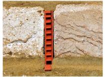
Weep vent to allow the transit of water, to expel onto outer wall, to maintain a dry cavity.
